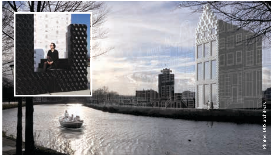
A rendering of the Canal House. Inset: the house's building blocks, forged by a 3D printer.
